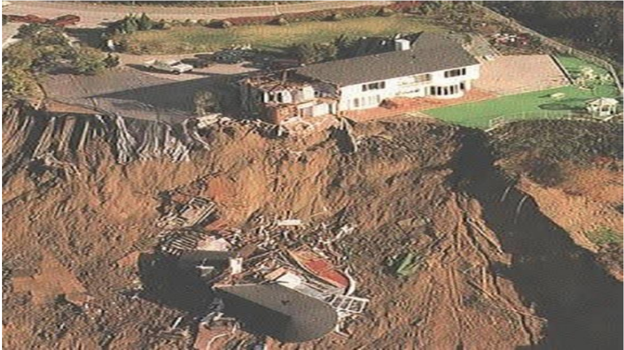
Figure 14 – Landslides and slope buckling under residential buildings from the 1994 Northridge, California, USA earthquake.
