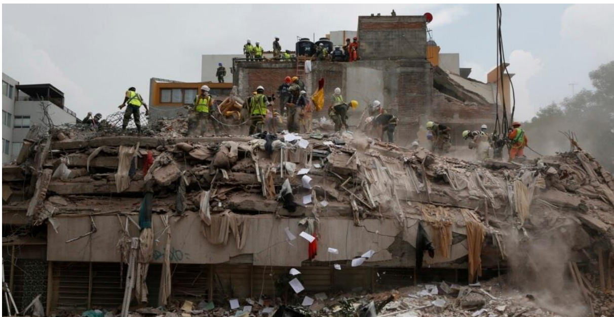
Figure 10 – Collapsed building as a result of the 2017 earthquake in Mexico City, Mexico.
